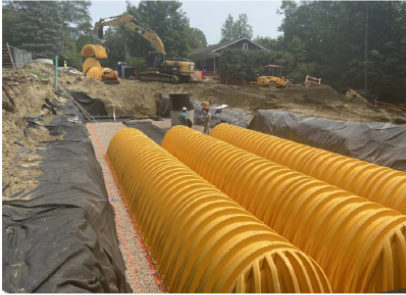
Dry Wells and Detention Chambers
